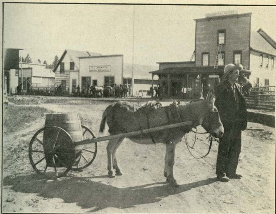
HAZELTON MAIN STREET. SHOWING THE WATERWORKS SYSTEM.
